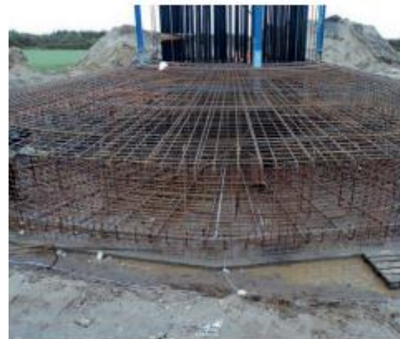
Figure 3 Reinforcement of a wind turbine with foundation earth electrode
