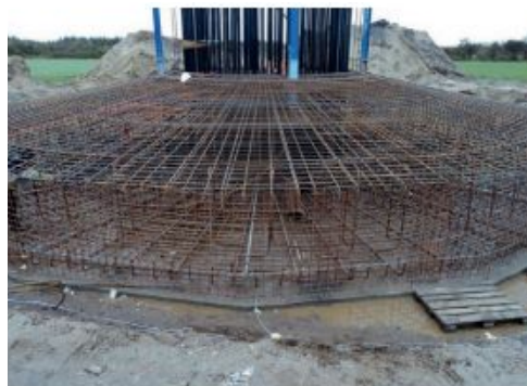
Figure 3 Reinforcement of a wind turbine with foundation earth electrode
